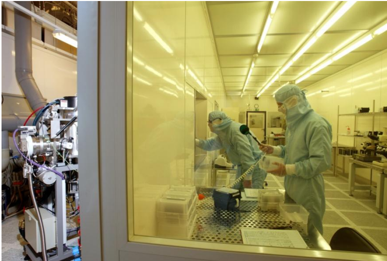
Bay and Chase Cleanroom Arrangement
